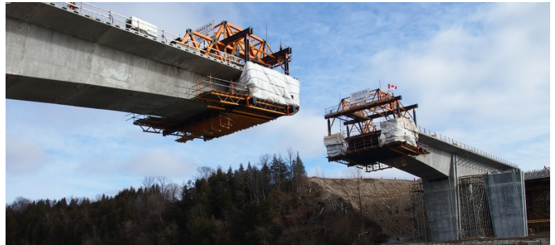
Figure 25. Construction on the Fairway Road Extension.
