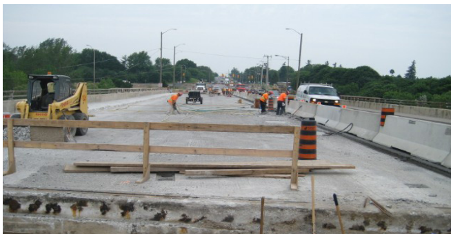
Figure 26. Highway 7/8 Construction in Kitchener.
