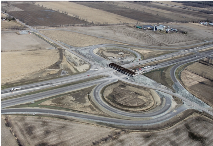
Construction on Highway 7 Source: Government of Ontario. (2011).
